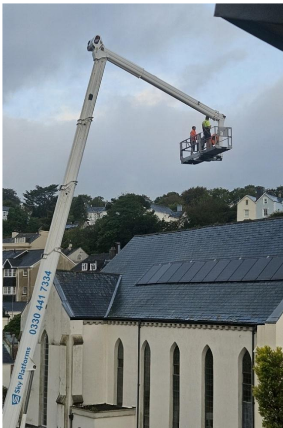
‘Intervention from on high!’ - Work on the roof of our Church last month. Photo from Anne Snook.
